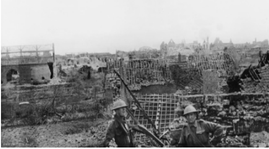
Shattered buildings in the French village of Lagnicourt, which was captured by the Australians in late March 1917 as the Germans withdrew towards the Hindenburg Line. The Germans heavily shelled the village as they retreated.
